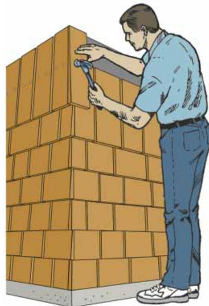
Figure 9: Fitting Laced Corner Courses
